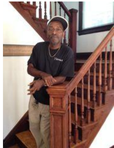
Eric Standifer, of M&M Construction & Remodeling, Walnut Hills, displays the restored wooden staircase of the home at 3561 Bogart Ave., Avondale. (Photo: Mark Curnutte/The Enquirer )
