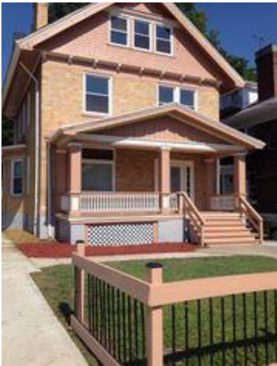
In one year, several investment partners in Avondale remodeled the house at 3561 Bogart Ave., near the Avondale Town Center, which will be dedicated Friday night with a ribbon cutting. (Photo: The Enquirer/Mark Curnutte )
